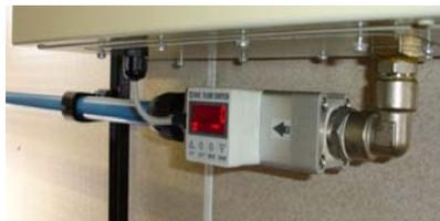
Breathing air flow is displayed and monitoring prevents system shut down while it is supporting life.
