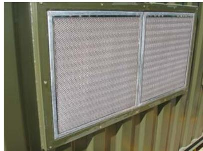
Stainless steel salt filters protect the equipment in coastal locations.
