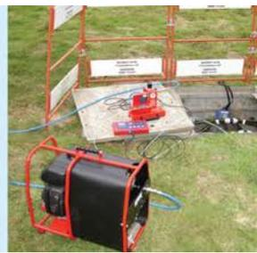
The 4A is the next generation in blown fibre technology for installing EPFU – enhanced performance fibre unit. Incorporating an extremely efficient air delivery system the unit is designed to use significantly less airflow compared to other blowing heads. As a result this allows the unit to blow to the same standard with considerably smaller air compressors, such as the petrol engine driven BT9A or Factair's 110/240V Electric Blown Fibre Compressor, which both weigh under 25Kg.
